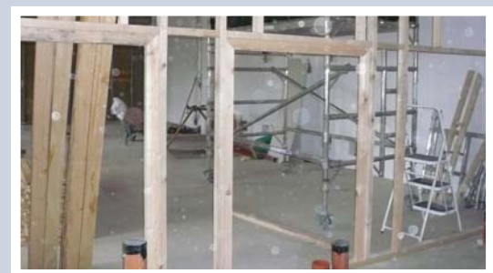
Putting in the barrier wall
