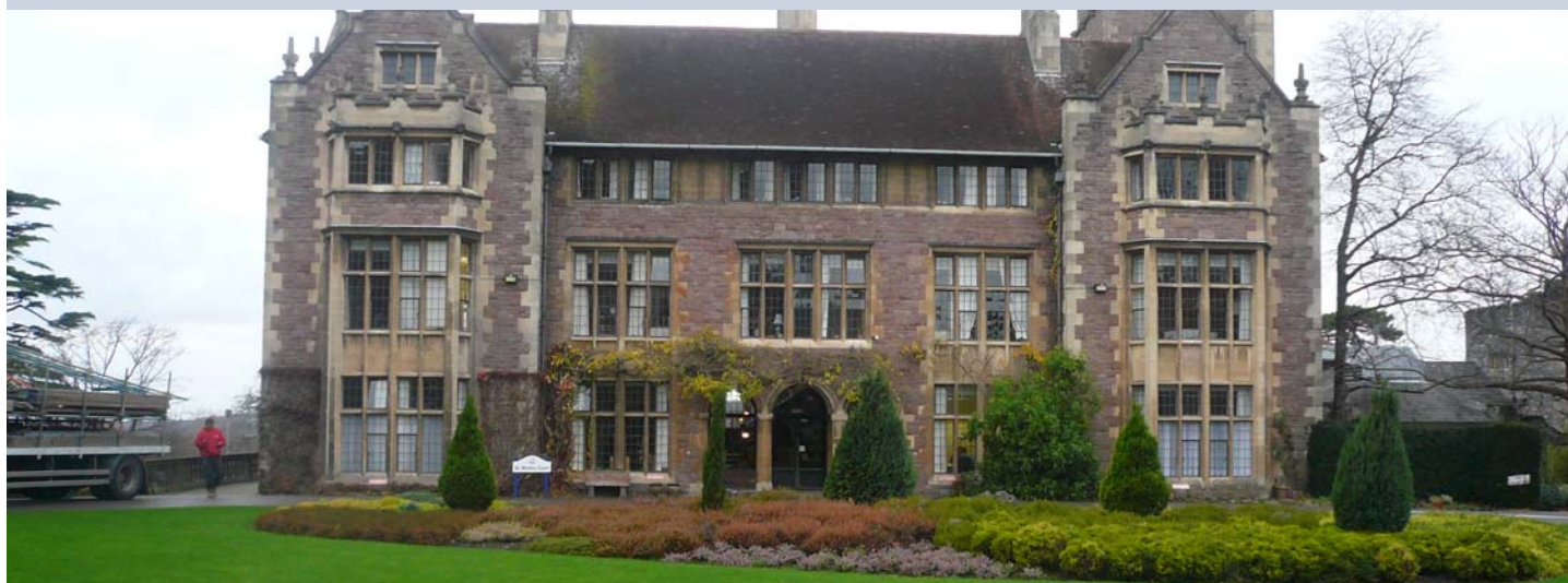
One of the beautifully maintained listed buildings at the Cote Lane site
