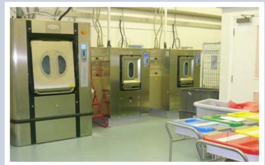
The dirty side with the three barrier washers. Towards the right is the door to the refrigerated room for weekend storage.
